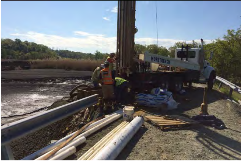
CCR Impoundment Closure - Dewatering
